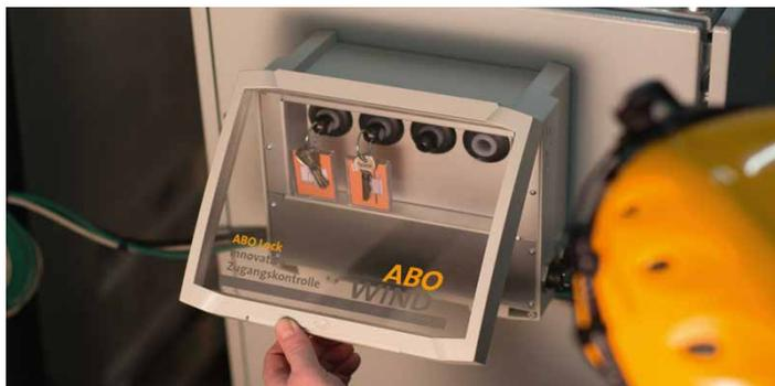
All keys, e.g. for the service lift, transfer station or the medium-voltage switchgear, are electronically secured in the key management system.
